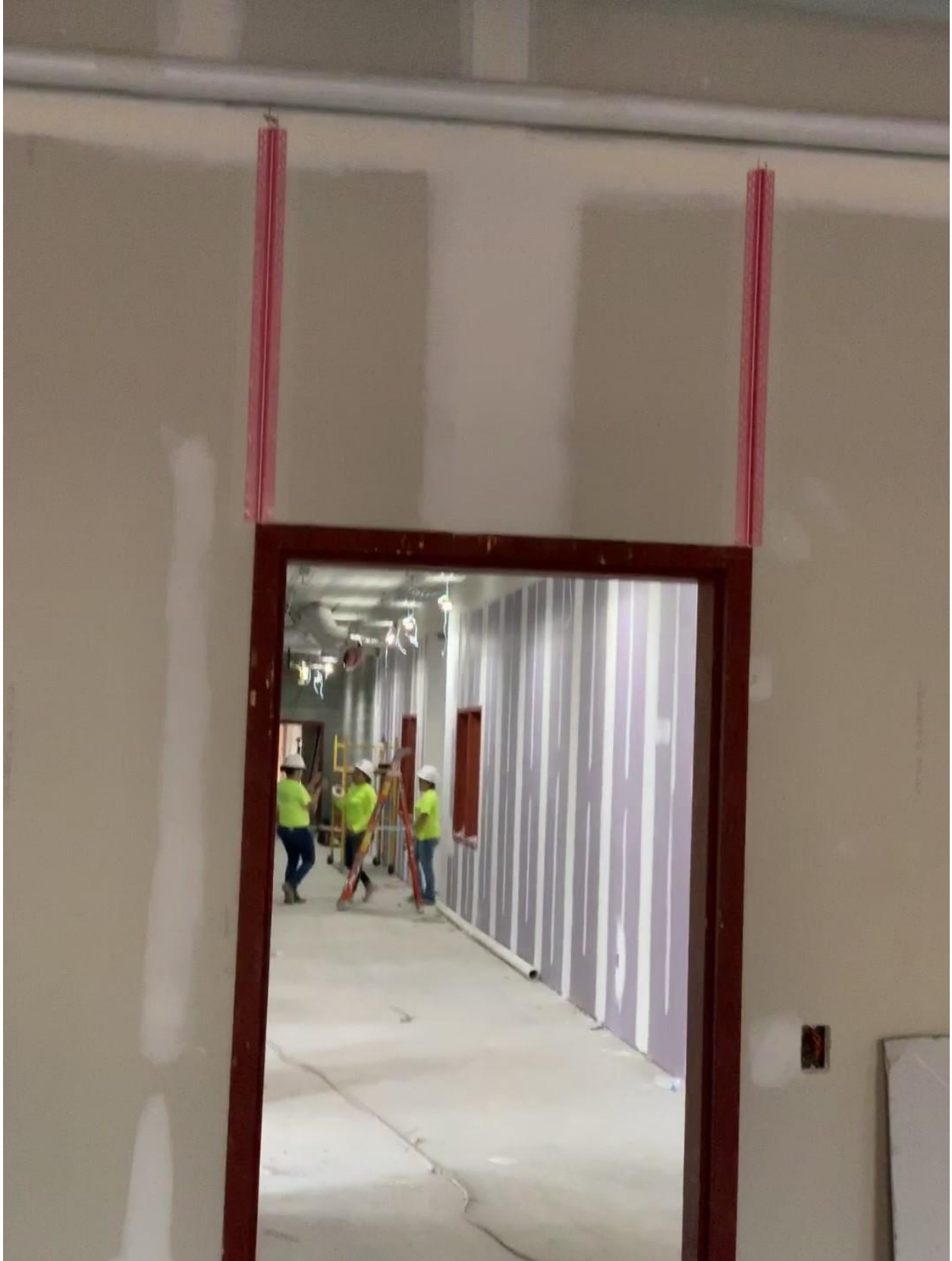
This is where the drawings call for the sheetrock to be grooved to keep cracks
