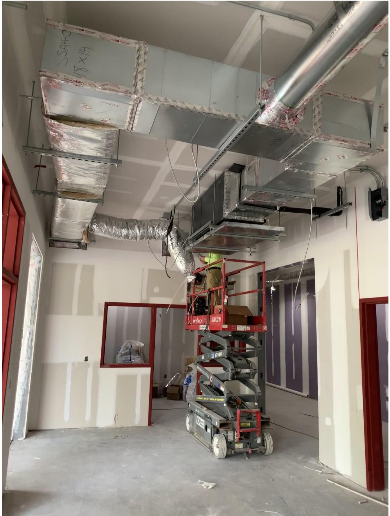
Work is taking place throughout the new construction but it takes a lot of looking
